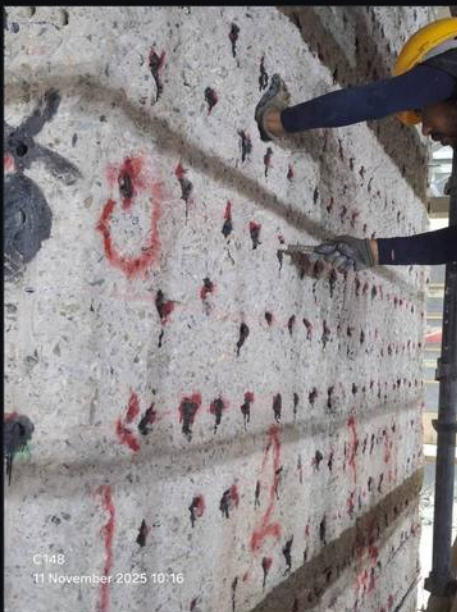
C148 • 11 Nov 2025. Weak concrete removed, substrate roughened, anchor grid set out and primed – step one of five.
