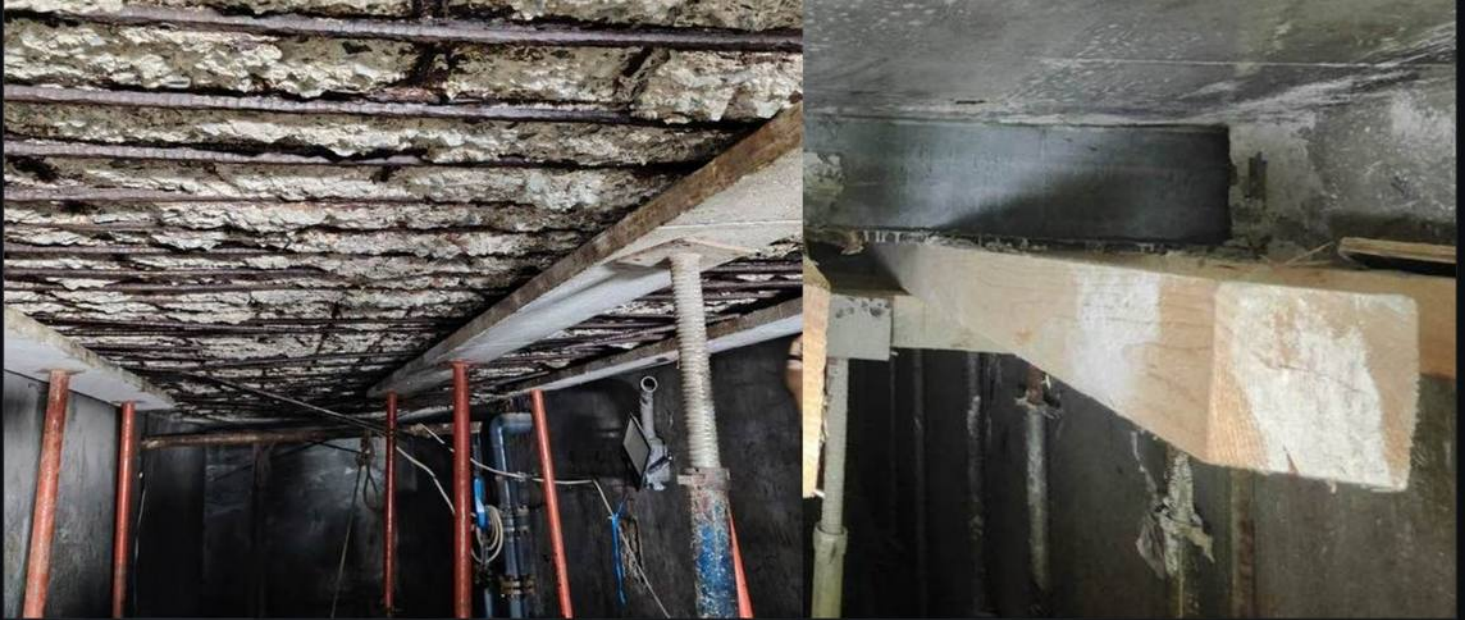
The tunnel, one month apart – drag the handle. Section loss across the full width of the soffit, cover concrete removed for inspection; new steel support installed, secured, and the soffit made good.
