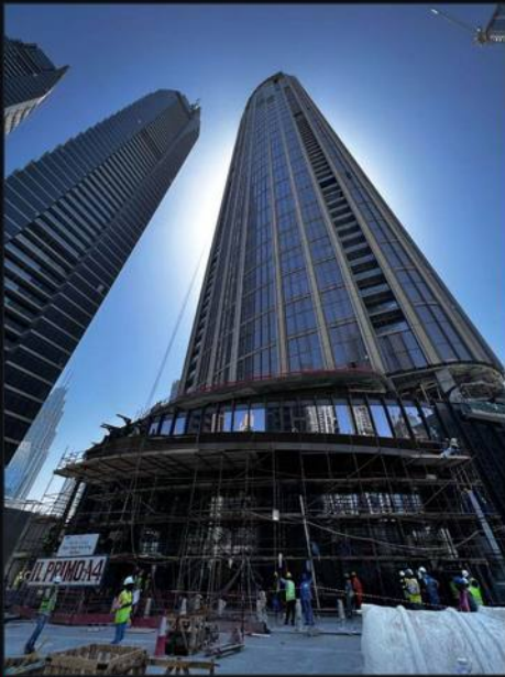
Il Primo, from the site. 356 m at topping out.
